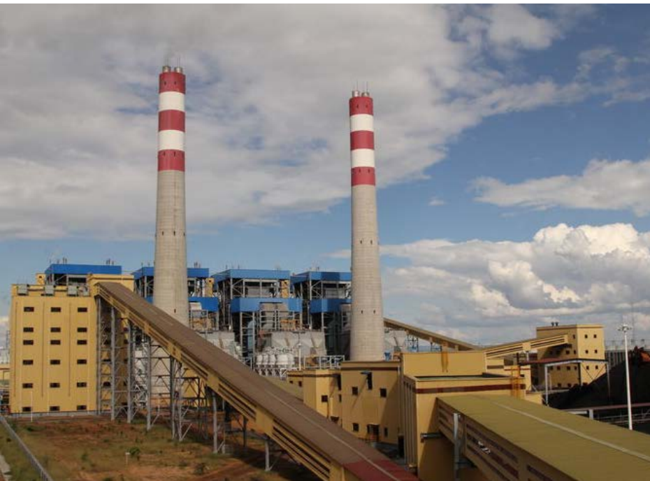
Morupule B power station, Botswana
