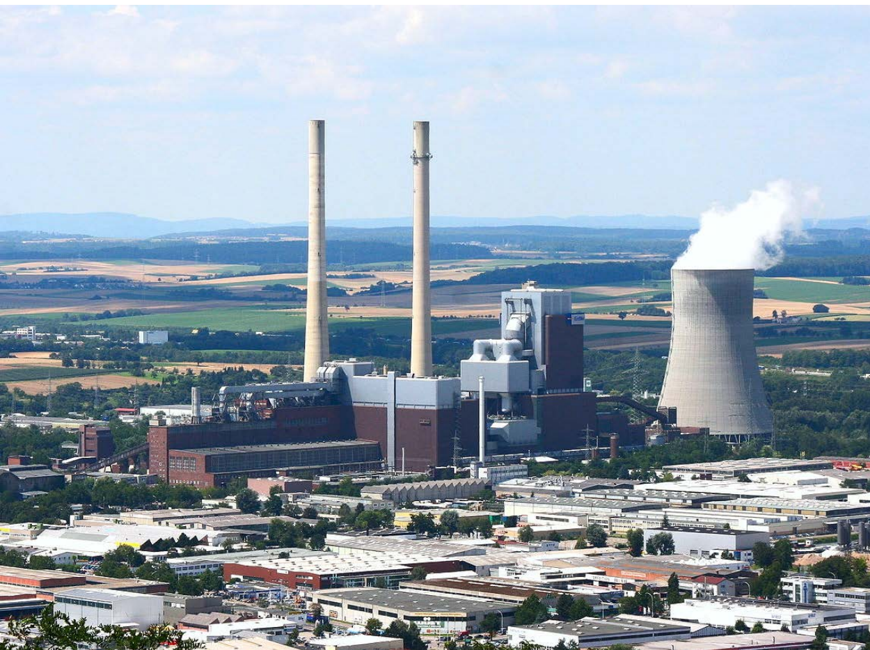
Emsland natural gas-fired power plant
